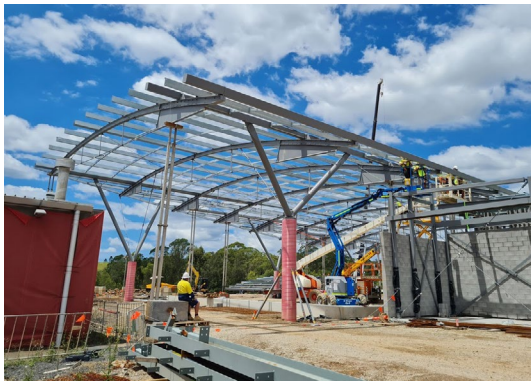
Construction of the fly-roof for the new Herbarium. Photos: courtesy of Hannah McPherson.
