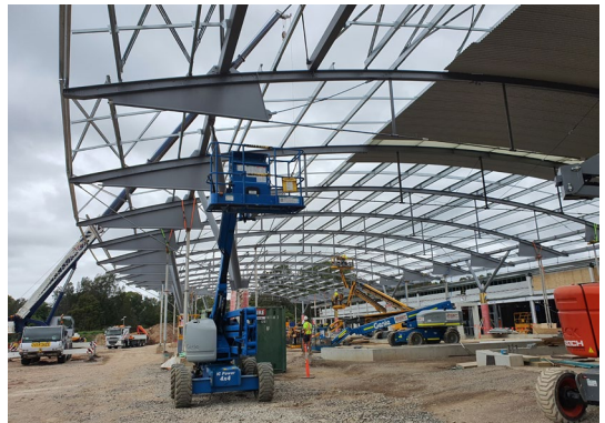
Construction of the fly-roof for the new Herbarium. Photos: courtesy of Hannah McPherson.
